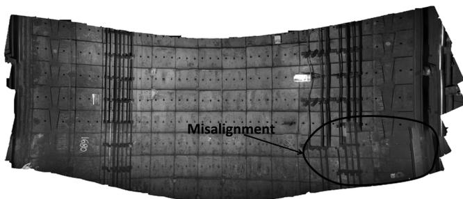
**Fig. 18.** Result obtained from Bond Street Station is created from 123 images and covers 7 m in the longitudinal direction
