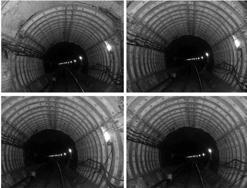
**Fig. 4.** Pictures of tunnels from the Aldwych site obtained by forward motion; only small parts of the tunnel surface are visible in these images, making them unsuitable for inspection
