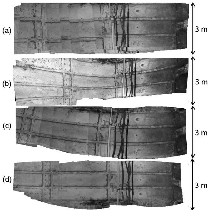
**Fig. 17.** Results obtained from the Aldwych data set: (a) mosaic before the BA algorithm is applied; (b) typical result from commercial stitching software; (c) result obtained from the experiment when an incorrect surface proxy is used for mosaicing; (d) final result obtained from an accurate surface proxy
