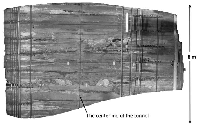
**Fig. 2.** Result created from the proposed mosaicing system that preserves all physical attributes, e.g., line parallelism and straightness, which are important for tunnel inspection; the mosaic was constructed from 173 images
