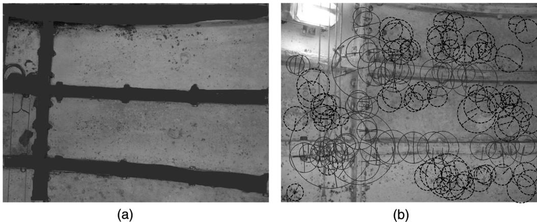
**Fig. 11.** (a) Example of a labeled image for SVM training and testing, the nonsurface region is colored in dark grey; (b) the points in solid grey lines and in dotted black lines are estimated as the nonsurface class and the surface class, respectively
